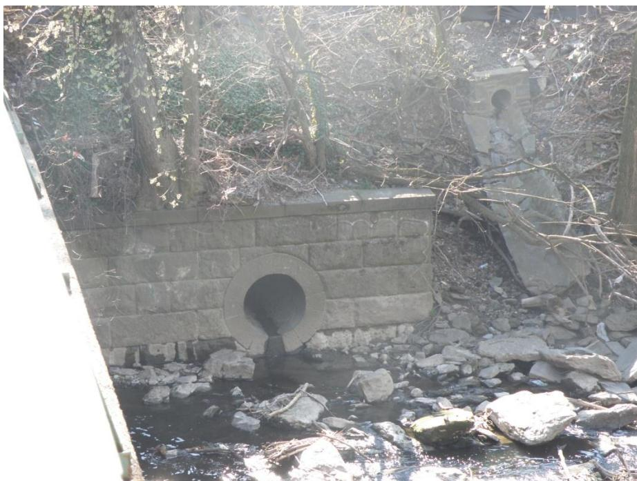
Left wing wall with pipe passing through it. Also note downstream pipe with undermining of concrete channel
