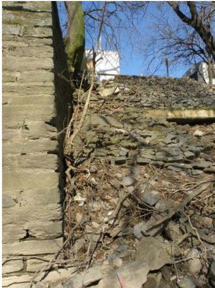
Undermined rock slope protection
