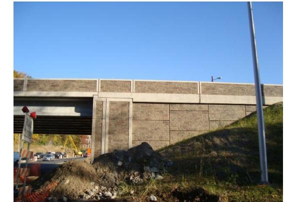
Concrete formliner and staining on adjacent Lincoln Drive Bridge.
