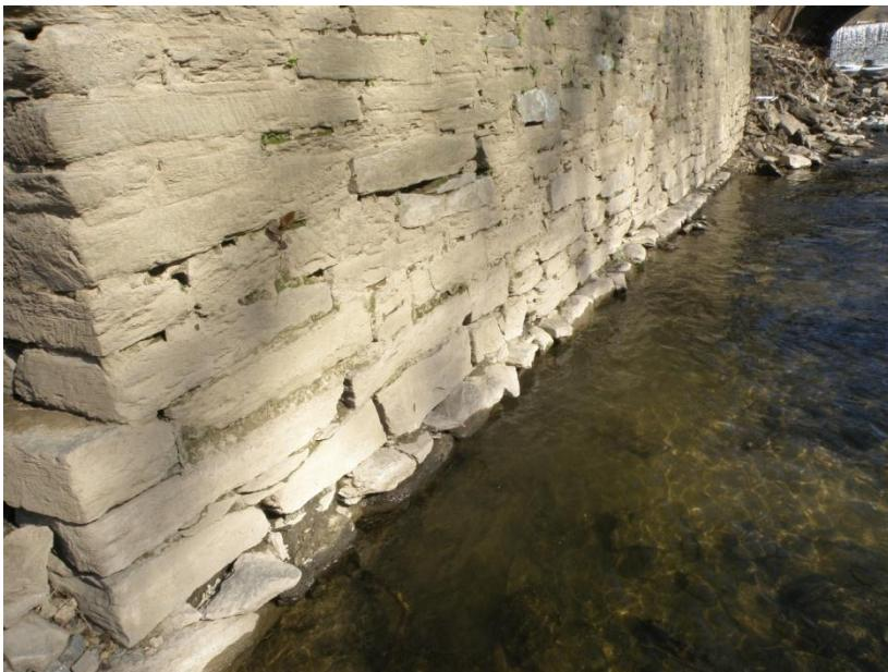
Foundation stones at right abutment. Note mortar loss particularly in the lower courses.
